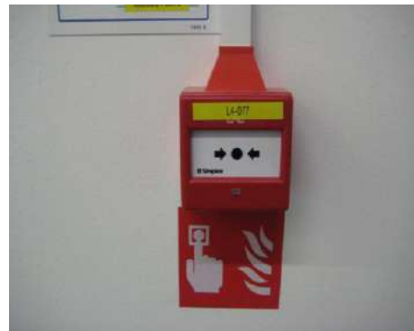
Types of break glass units found above in the Terminal building
