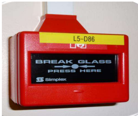
Types of break glass units found above in the Terminal building
